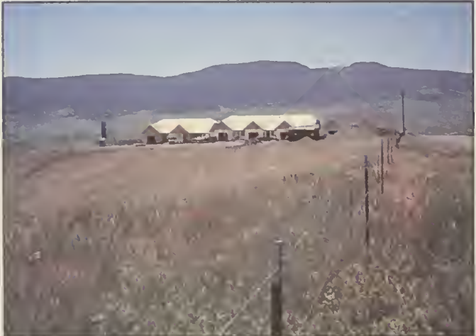
New construction on a reclaimed gravel pit.
